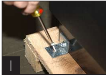
1 Removing bracket from skid.
