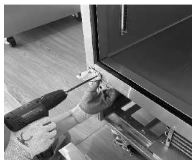
F. Assemble the bottom hinge
