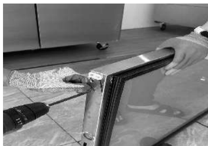
D. Disassemble the stopper plate, then tight screws
