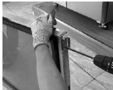
E. Assemble the stopper plate in original positions
