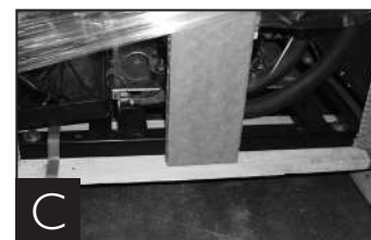
Removing skid from bottom of cabinet.
