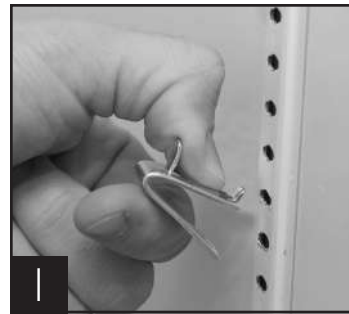
1 Installing top tab of shelf clip
