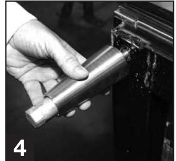
4 Thread leg into cabinet bottom frame rail.
