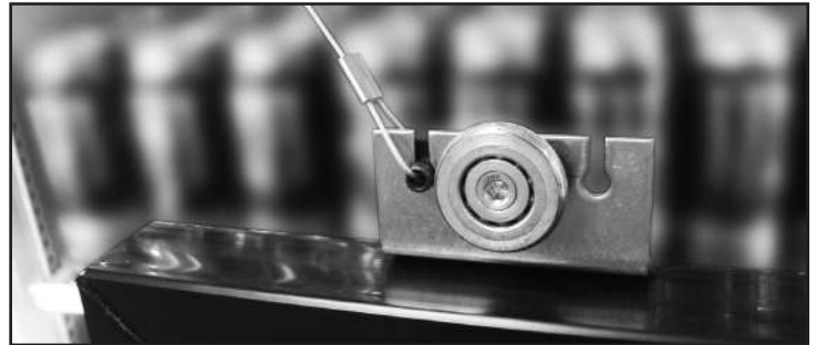
Fig. 9. Be sure the door cord is in the roller slot closest to the pulley.
