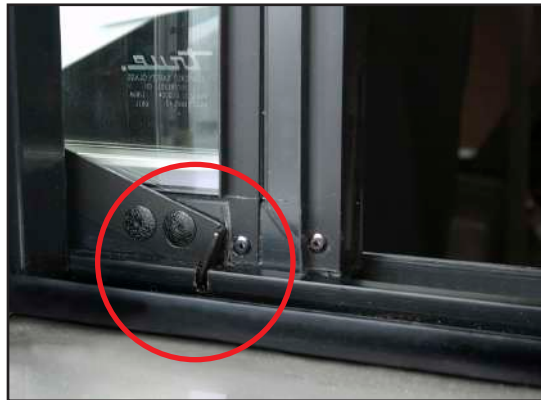
Fig. 1. Door latch is in the open position (engaged with notch).
