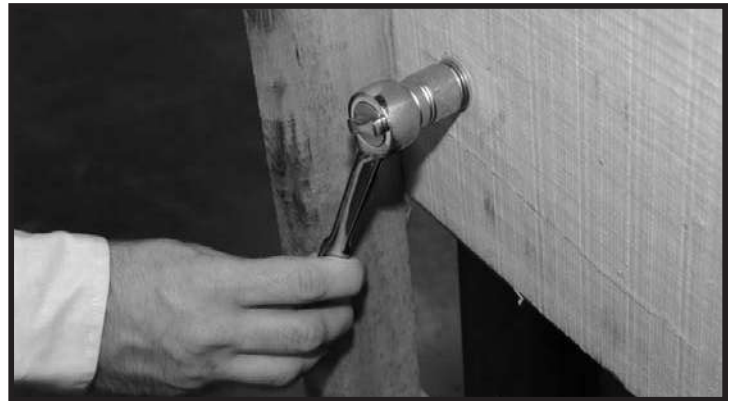
Removing skid from bottom of cabinet.
