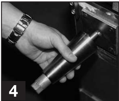
4 Thread leg into cabinet bottom frame rail.
