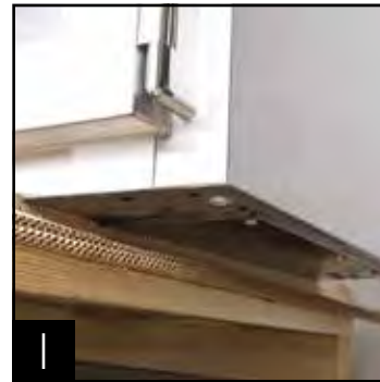
Slide packing material under the unit.
