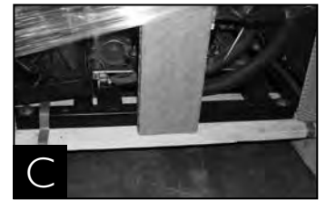
Removing skid from bottom of cabinet.
