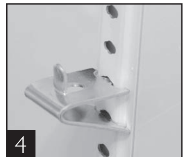
Shelf clip installation complete
