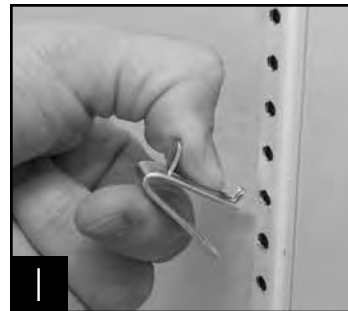
1 Installing top tab of shelf clip
