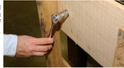
Removing skid from bottom of cabinet.
