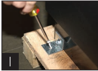
Removing bracket from skid.
