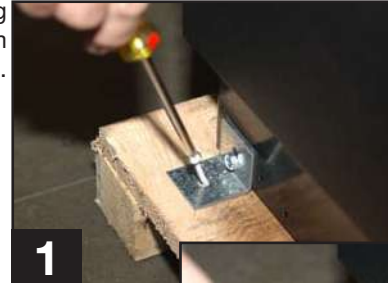
Removing bracket from cabinet.
