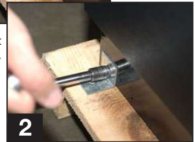
Removing bracket from cabinet.
