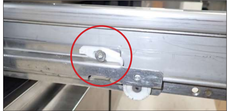
Fig. 1. Drawer retainer location. Retainer is engaged.
