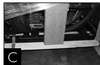
Removing skid from bottom of cabinet.
