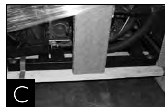
Removing skid from bottom of cabinet.
