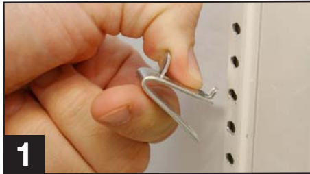
1 (Installing top tab of shelf clip)
